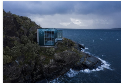
Located in the village of Skutvik, Norway, the striking modern structure for the Arctic Salmon Center is clad in panels that create the illusion of Nordic salmon scales. Photo courtesy Steni
